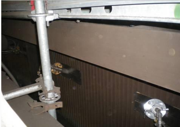
Left Boiler Wall
