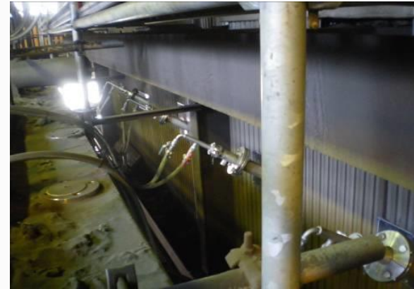
Right Boiler Wall
